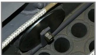
When cleaning exchanger pipes (pic.3/23) make sure that flap area is clean, as well as flap itself (pic.3/15). Flap leakage can decrease boiler power.
