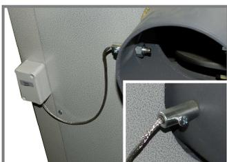
For proper operation of exhaust gas thermometer is very important its cleanliness. When cleaning heat exchanger always gently wipe away dust from thermometer.
